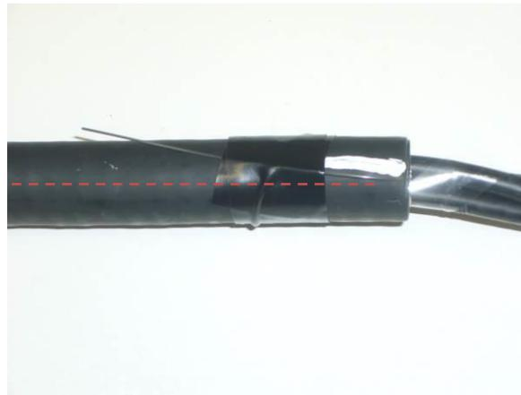
As an additional safety measure (and in case the mark is not visible) the installer should cut circular through aluminium armor and jacket approximately 30 cm away from the end. Then he should move this piece of armor approximately 2 cm towards the F/O connectors. Through this “window” he can easily verify the neutral position of the ripcord. Observing this neutral position he can now cut in one step through the loose and the fixed part of the armor/jacket.
